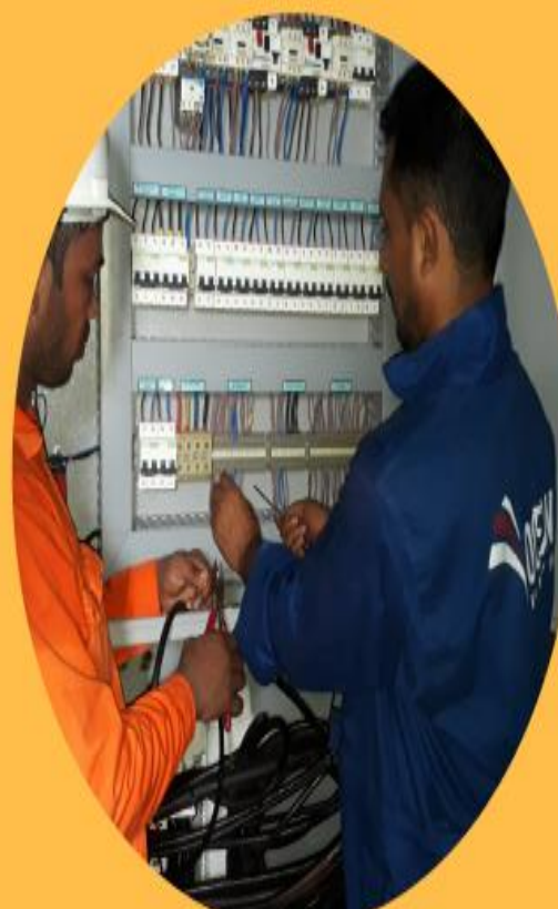
Cable Pulling & Termination onboard
