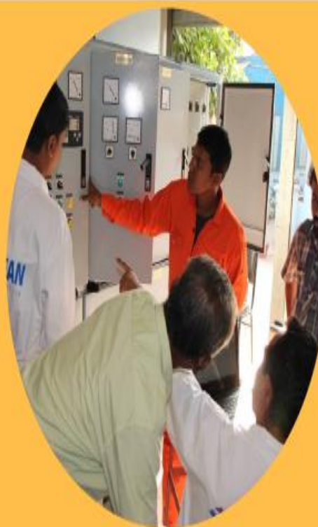
Factory Acceptance test of Switchboard under class
